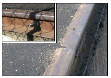
Old rail used as edging for the trackside platform has been bolted in place and holes in the asphalt filled in.
