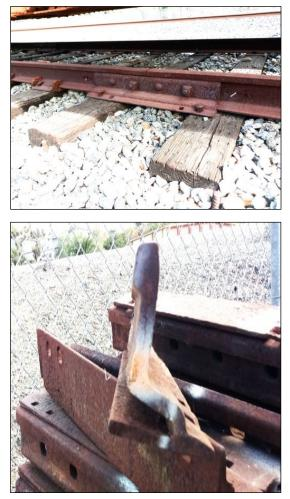
Museum volunteers struggled to salvage the shelf-type bars and to fit them onto the rails while building the display track, requiring more precise alignment than typical joint bars. But they provide more support and spiking options where rail ends do not occur above the wood tie. Such bars are no longer used because spiking near tie edges caused splitting, and skewing ties could cause narrowing of the gauge.
